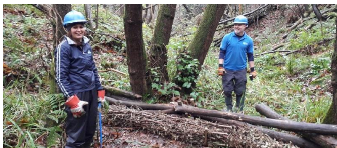
Figure 10: Volunteers undertaking leaky dam work, ensure you have plenty cake (SFI).
