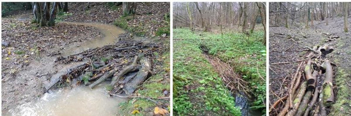
Figure 7: [Left] Gully stuffing in a flowing stream (SFI). [Middle] Brash bundles in a low lying woodland ditch (SFI). [Right] Gully stuffing in a steep, seasonally wet flow path (Stroud).
