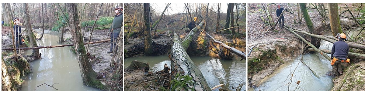
Figure 11: Contractors undertaking leaky dam work, utilising riparian trees as material for the leaky dams and as living stakes (Wild Sussex).
