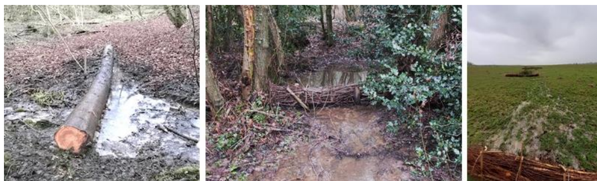
Figure 9: [Left] Log placed across flow path – note how water pools and spreads behind it (Stroud), [Middle] brush bundles across an overland flow path in woodland (SFI). [Right] brush bundle pinned across an overland flow path in pasture (SFI).
