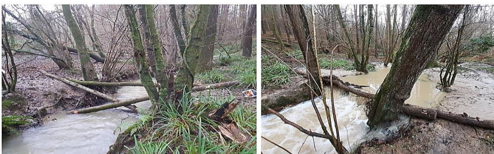
Figure 5: [Left] Looking downstream at a banktop diverter with a cross-shape within the channel. Pinned using rebar and riparian trees. [Right] Looking upstream at the same leaky dam during high flow conditions (SFI).
