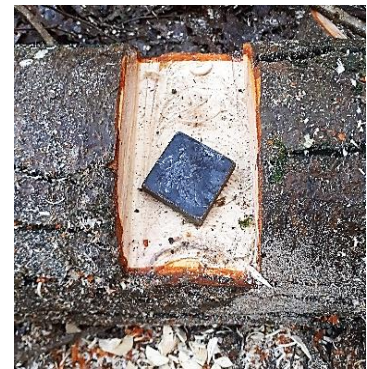
Figure 2: Rebar with a metal plate at one end, hammered through a log into the ground. A section has been removed from the log to ensure fixing is recessed (SFI).
